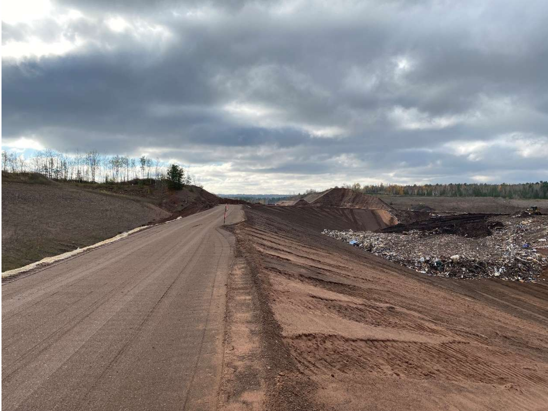
Location 9 – Looking south, Phase 6 eastern anchor trench
