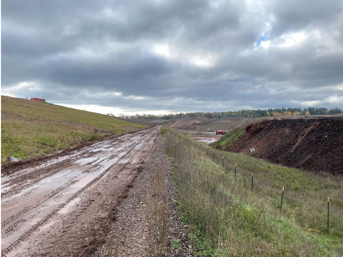
Location 4 – Looking South, Phase 3 Western Berm
