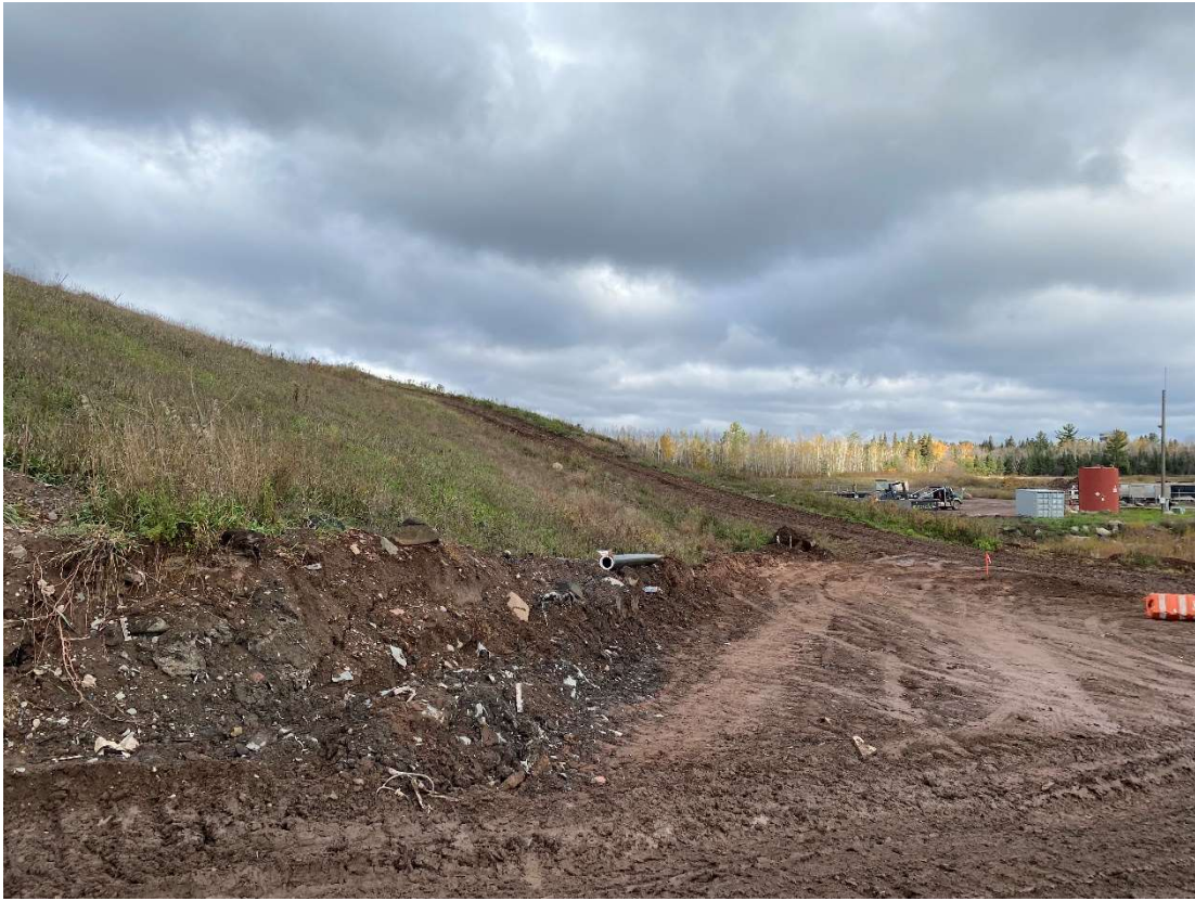
Location 11 – Looking North, Phase 1 anchor trench
