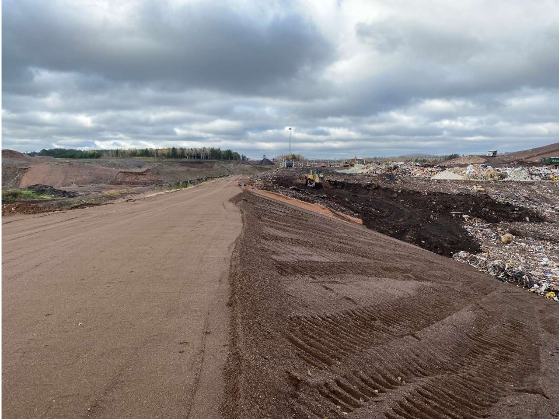
Location 8 – Looking West, Cell 6 Southern Anchor Trench
