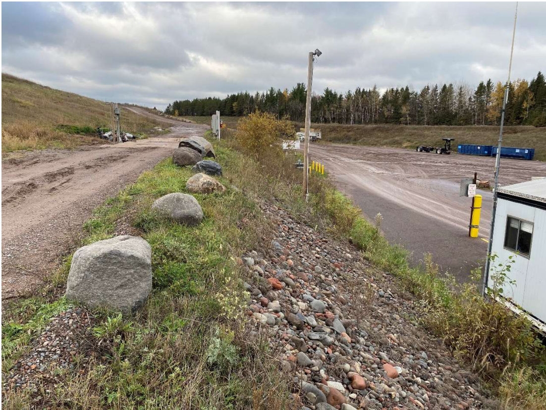
Location 1 – Looking West, Phase 1 Northern Berm
