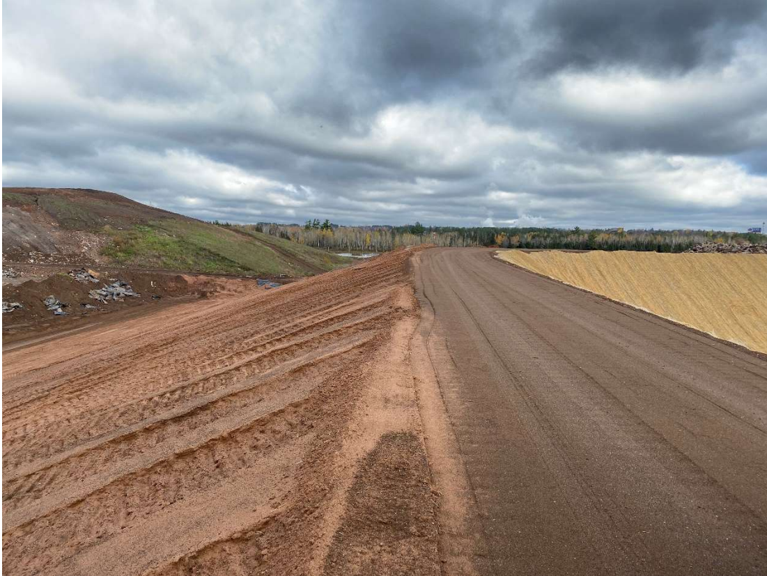
Location 9 – Looking north, Cell 4 eastern anchor trench
