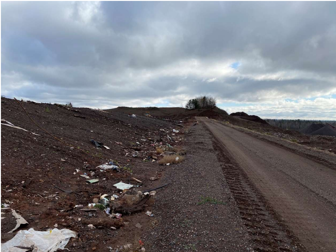
Location 7 – Looking East, Cell 6 Southern Anchor Trench
