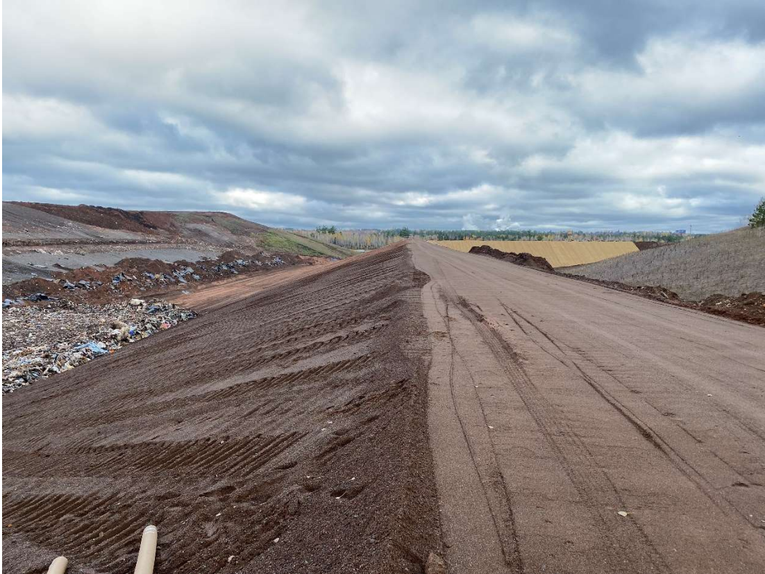
Location 8 – Looking North, Cell 6 Eastern Anchor Trench
