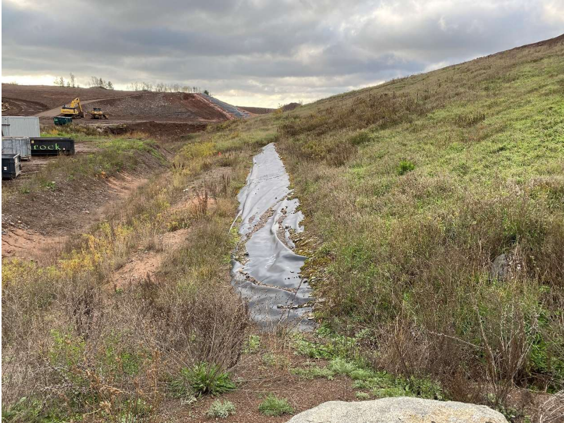
Location 1 – Looking South, Phase 1 Eastern Berm
