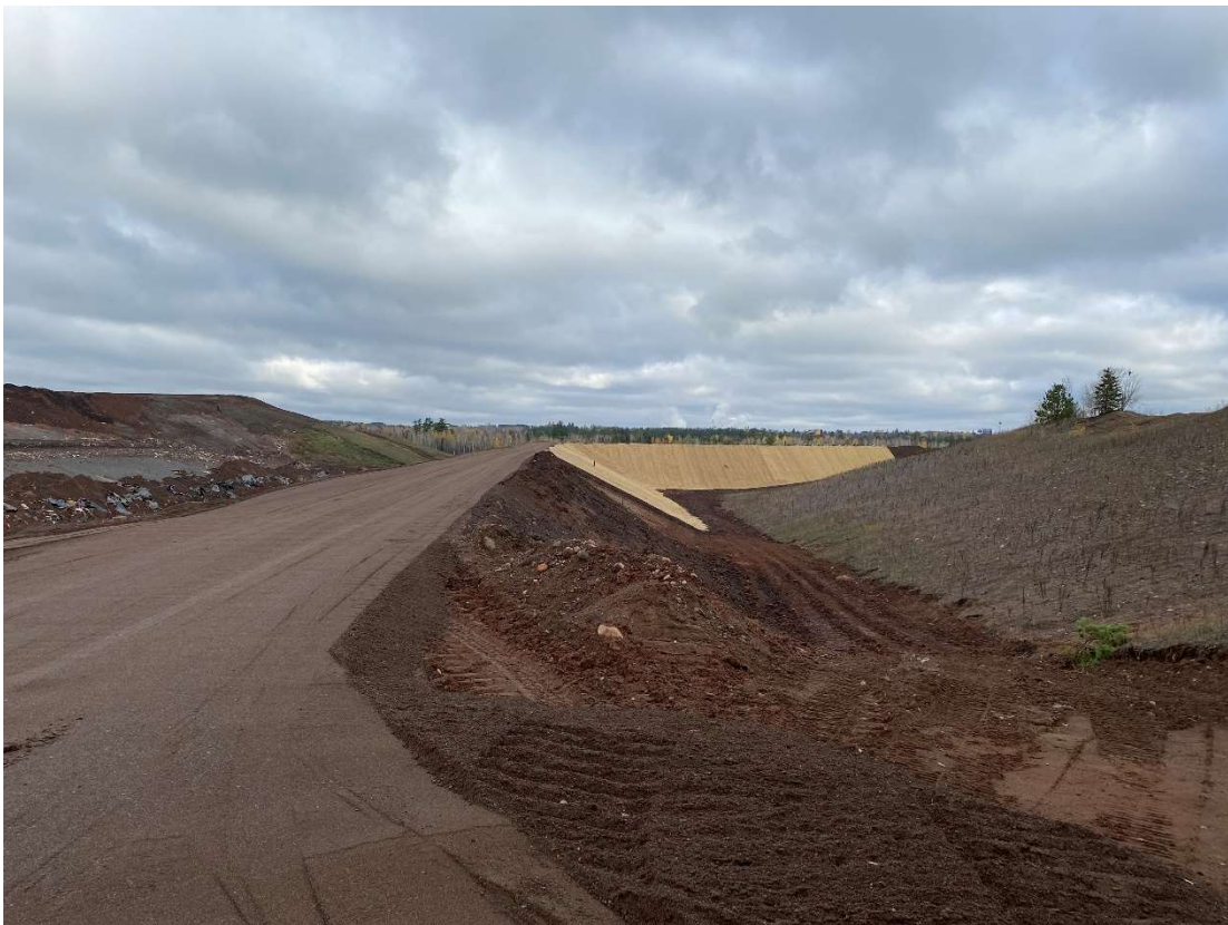
Location 8 – Looking North, Cell 6 Eastern Berm
