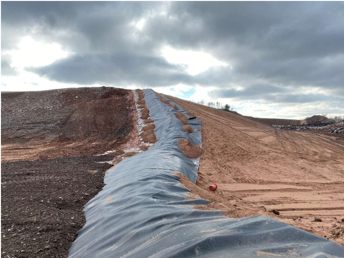
Location 11 – Looking Southwest, Phase 4 Southern rainflap
