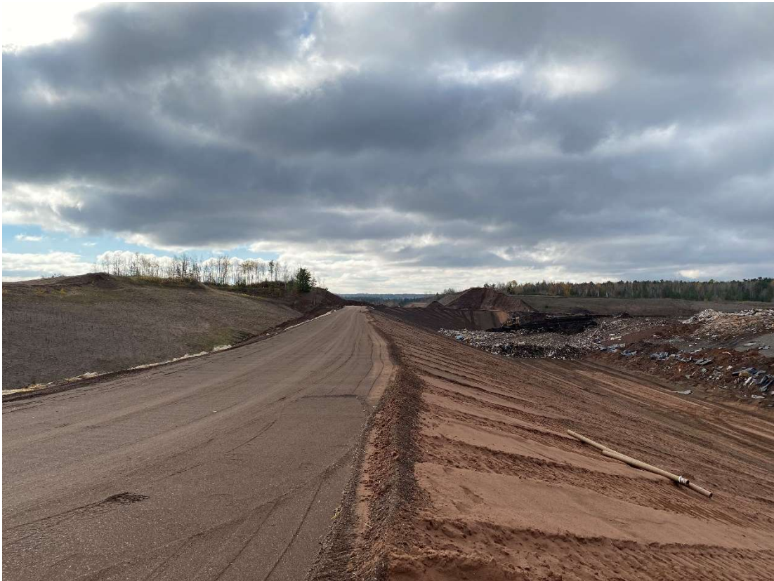
Location 10 – Looking north, Phase 4 anchor trench
