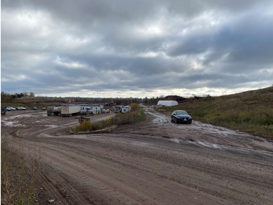
Location 2 – Looking East, Phase 1 Northern Waste Slope
