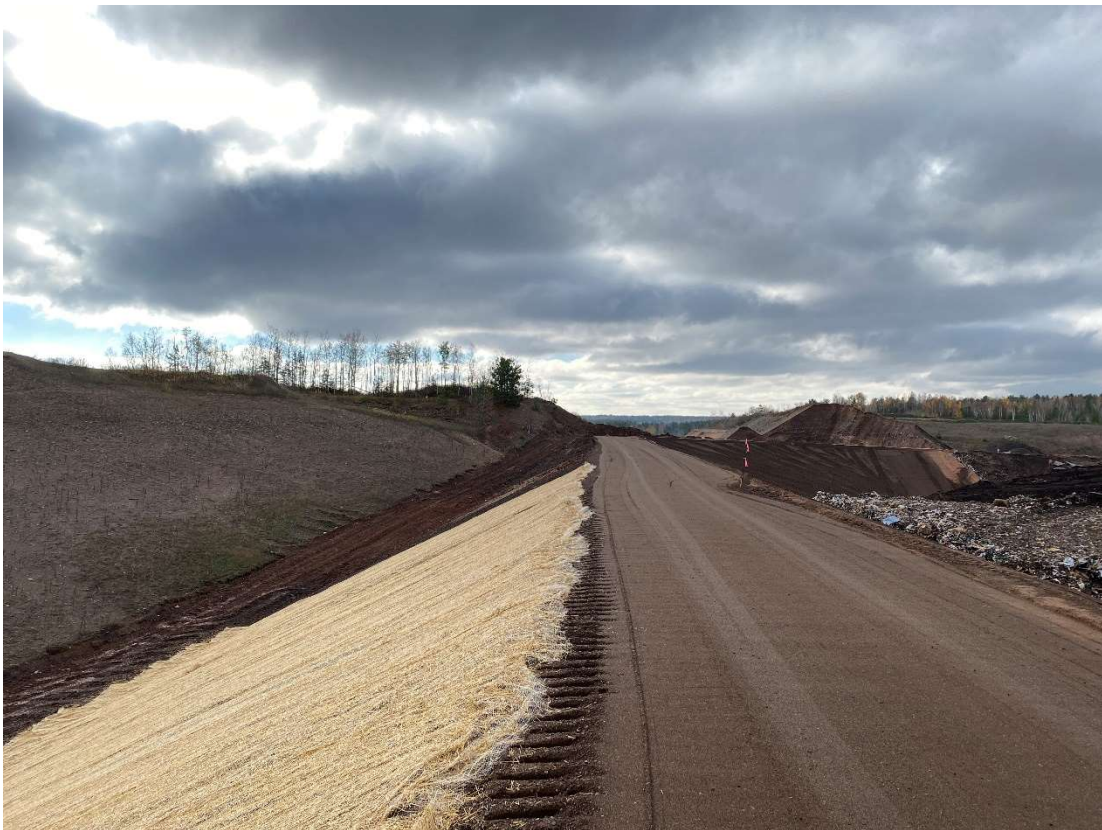
Location 9 – Looking south, Phase 6 outer landfill berm
