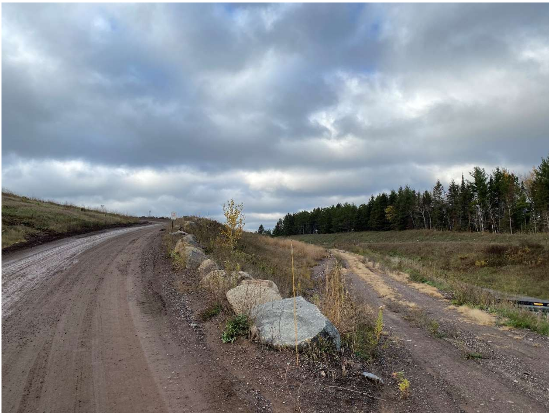
Location 2 – Looking West, Phase 2 Northern Waste Slope & Berm
