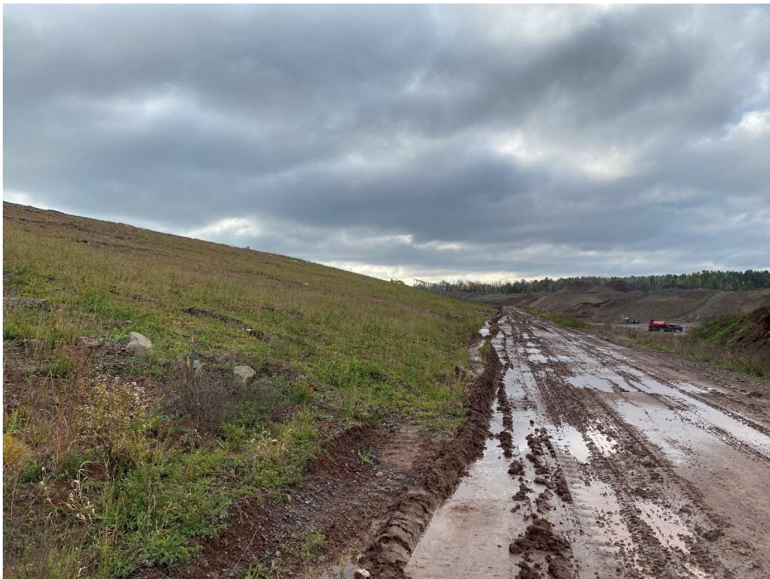
Location 4 – Looking South, Phase 3 Waste Slope
