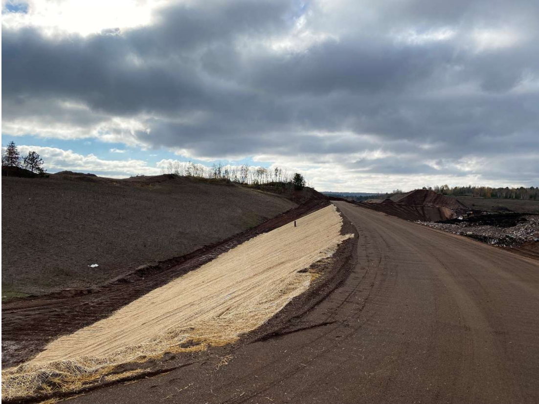
Location 10 – Looking north, Phase 4 outer landfill berm
