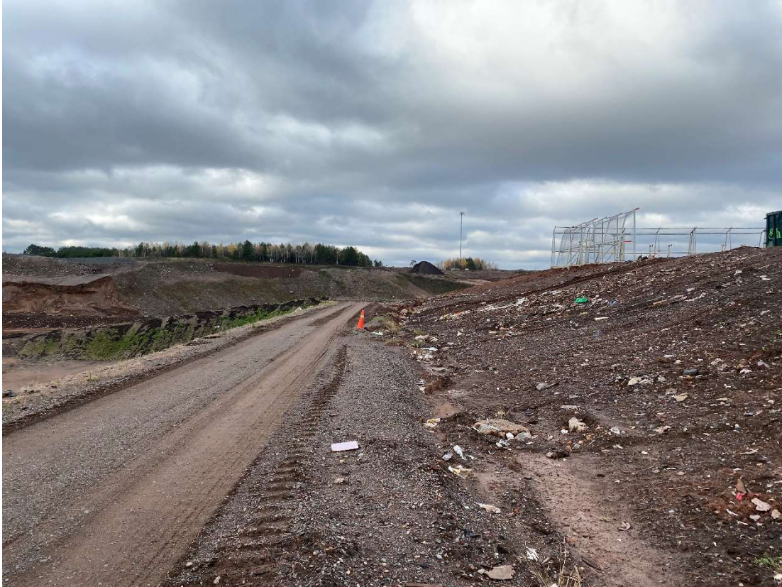
Location 7 – Looking West, Cell 5 Southern Anchor Trench
