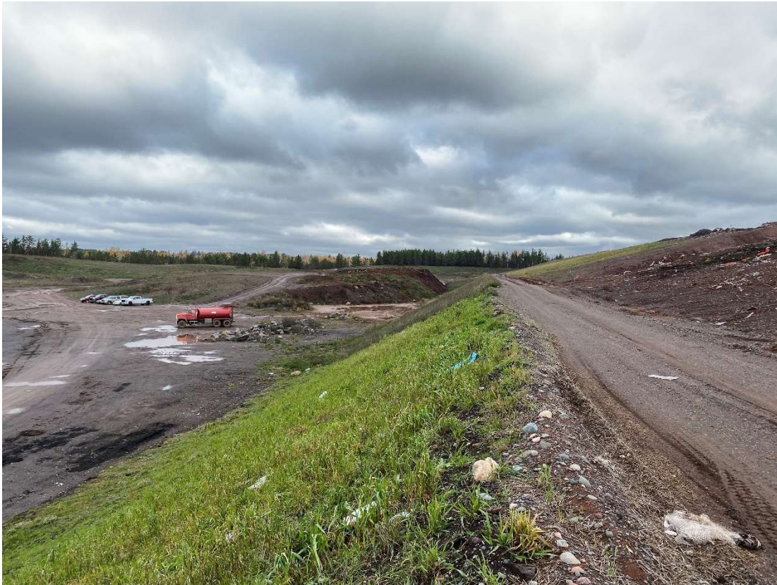
Location 6 – Looking North, Phase 6 Western LF Berm
